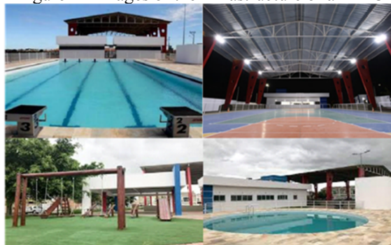
Figure 1 - Images of the infrastructure of an EEC
