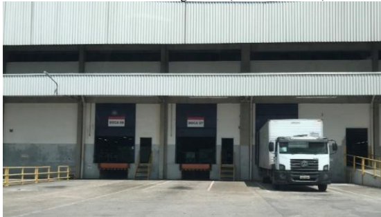
FIGURE 5 - Receiving Docks (Acai Warehouse)
