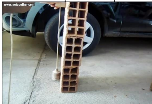
Figure 2: The use of the plume is to keep the wall upright.
