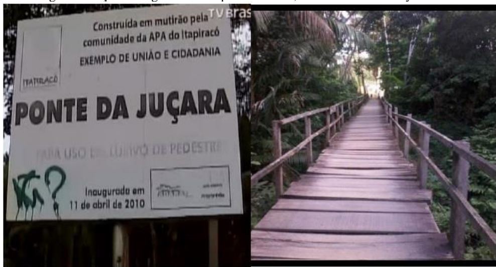
Figure 3: Juçara Bridge next to itapiracó stream, built in a community task force
