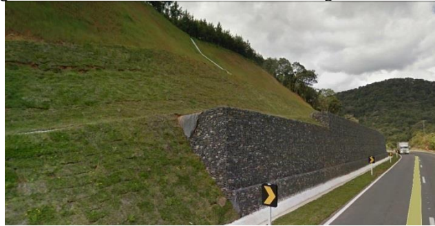
Figure 12. Containment structure - Retaining wall with rescan.
