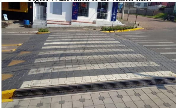
Figure 7: Elevation of the vehicle lane.
