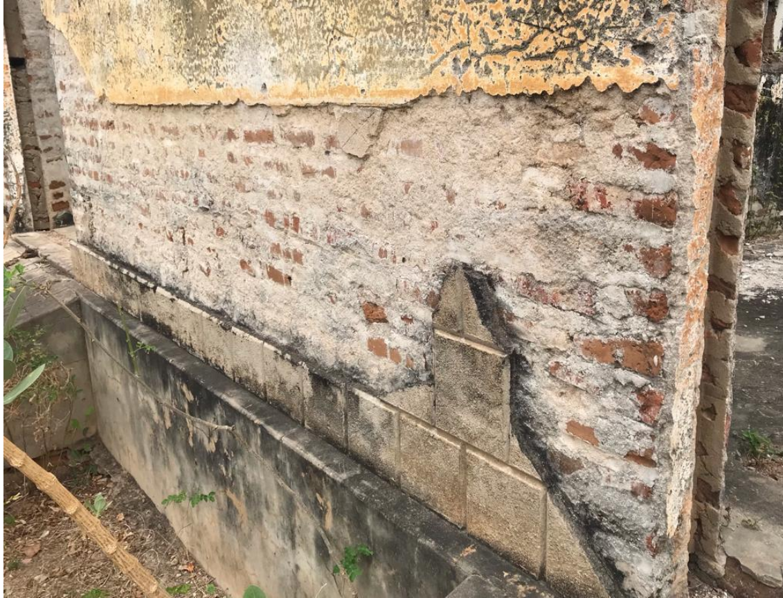
Figure 5 – Detachment of the mortar coating
