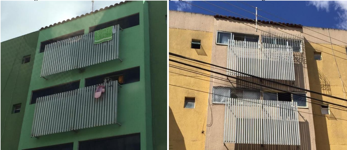
Figure 9 – Jirau: element on the facade for drying clothes with access through the service area.
