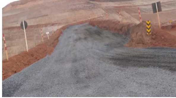
Figure 10. Improvement of access conditions with ceiling material.
