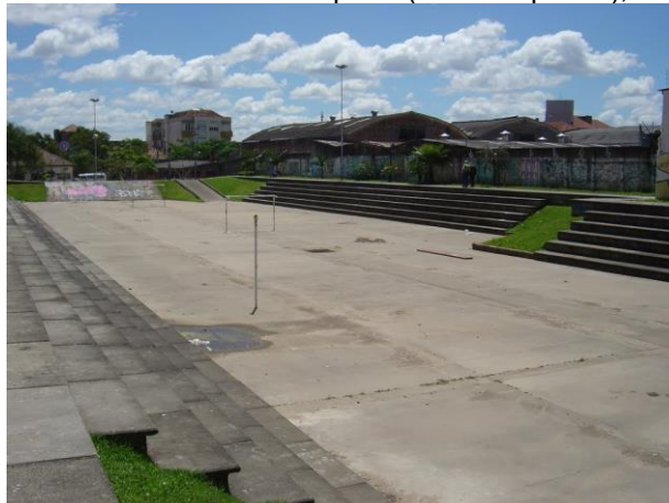
Figure 2: Detention Reservoir at Júlio Andreatta Square (Water Squares), Porto Alegre – RS - Adapted
