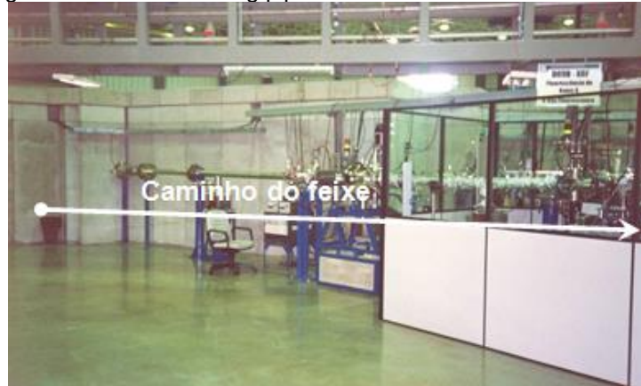
Figure 3: Photo of the ring pipe for the DO9B – XRF line of LNLS.
