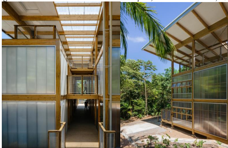
Figure 7: Photo of the internal and lateral façade, Author: Pedro Kok, 2018
