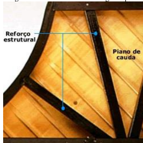
Figure 4: Structural beams of a grand piano
