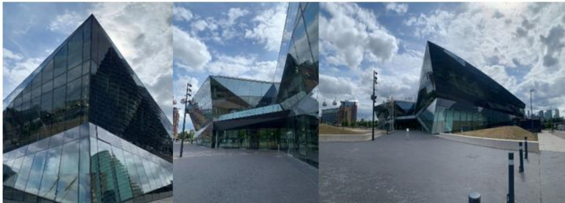
Figure 2: Exterior views of The Crystal building
