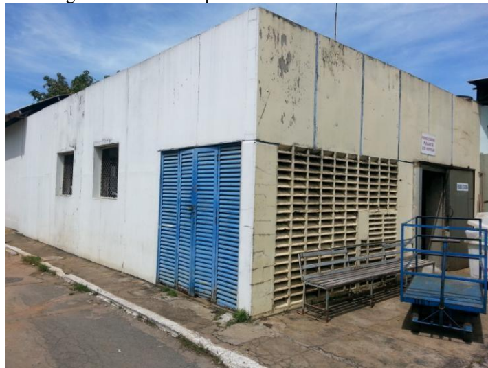
Figure 22 – Exterior photo of the current HRT shelter.
