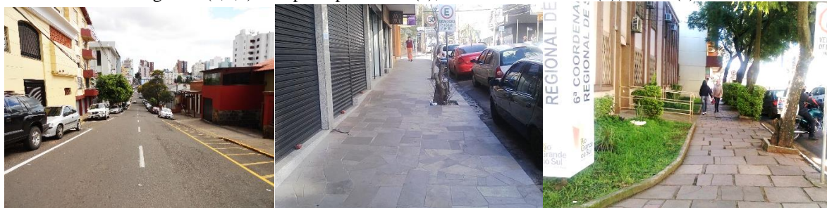
Figure 4 (a,b,c) – Asphalt pavement (a); Concrete Pavement (b); Lawn (c)
