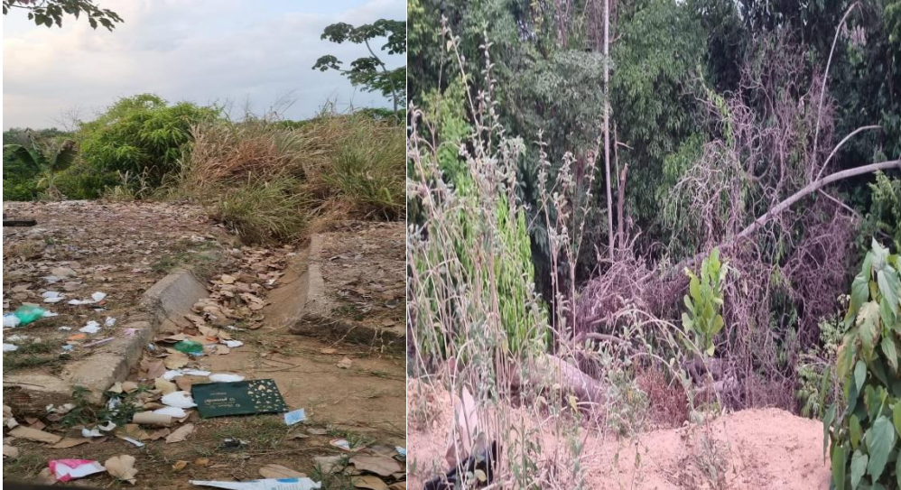
Figure 15: (a) maintenance-free duct system; (b) presence of erosion in the Colinas Park complex
