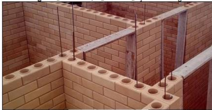
Figure 2 – Laying of ecological bricks
