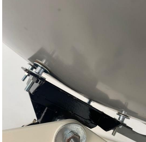
Figure 16 – Fixing structure of the offset dish.
