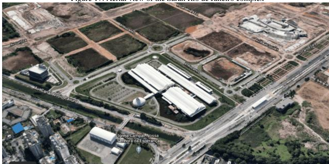
Figure 17: Aerial view of the Sarah Rio de Janeiro complex
