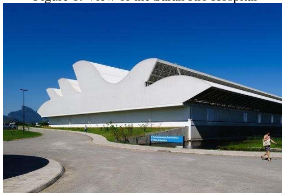
Figure 1: View of the Sarah Rio Hospital
