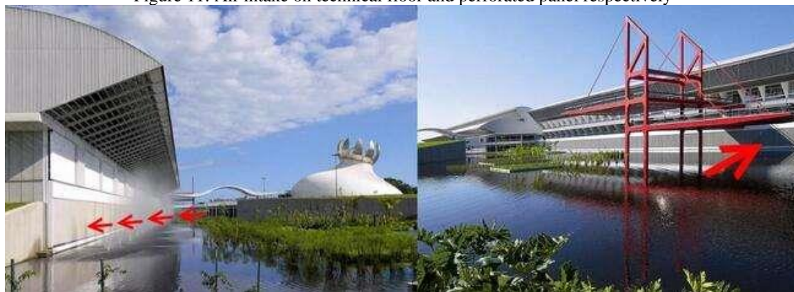
Figure 11: Air intake on technical floor and perforated panel respectively
