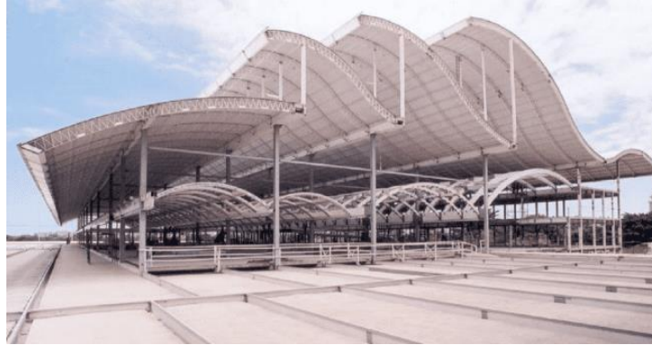
Figure 4: Rio de Janeiro's Sarah Roof Structure
