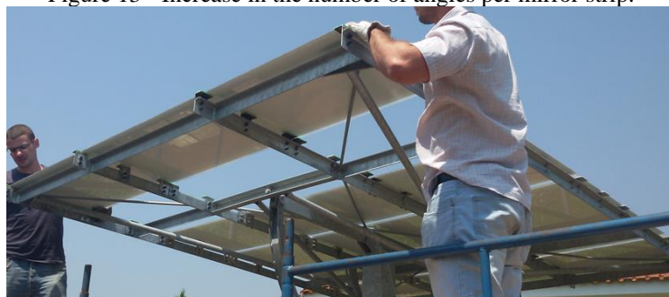
Figure 13 - Increase in the number of angles per mirror strip.
