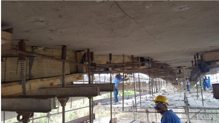
Image 3 - Of the shapes with the concreting
