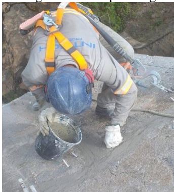
Cracks – sealing with grout. Source: Intech Engenharia (2016)
