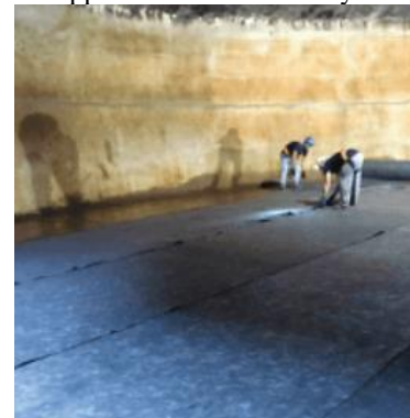
Waterproofing – application of blanket. Source: Tae Magazine (2020)
