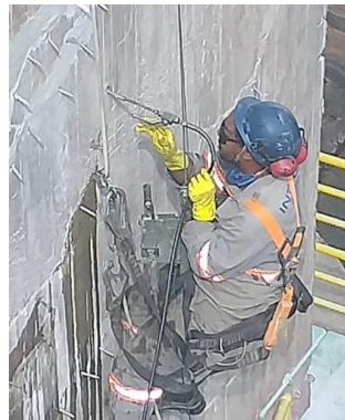
Cracks – injection of polyurethane. Source: Intech Engenharia (2016)
