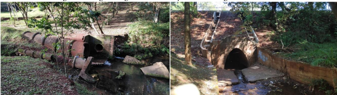
Figure 04: Engineering works in some points of the Água Fresca Stream.
