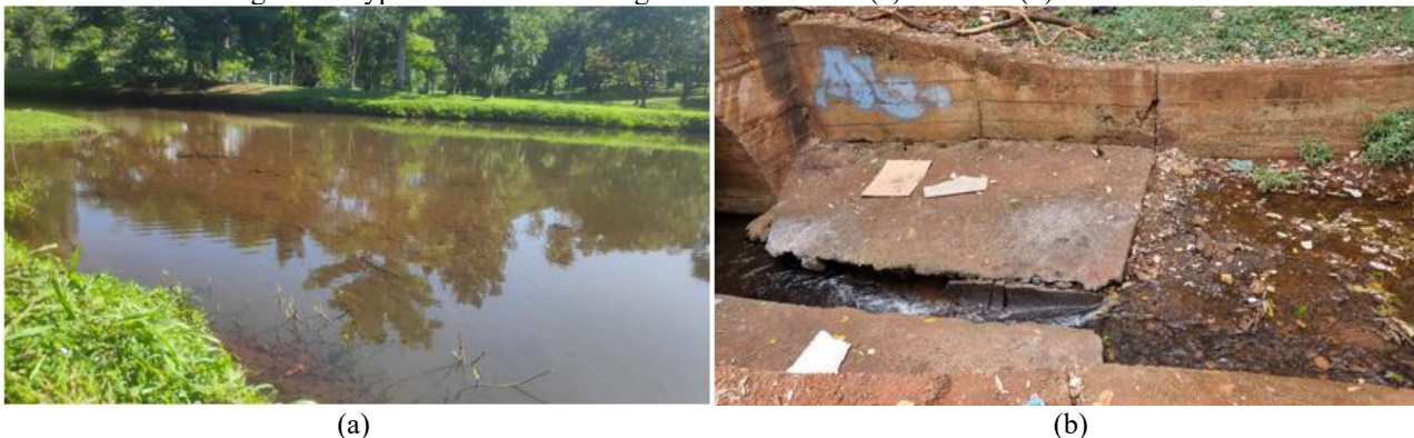
Figure 06 Type of bottom of the Água Fresca Stream: (a) mud and (b) channeled.
