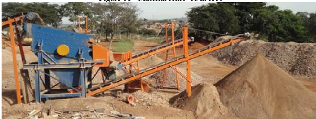
Figure 01 - Material removed in loco
