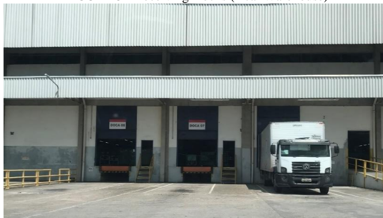
FIGURE 5 - Receiving Docks (Acai Warehouse)
