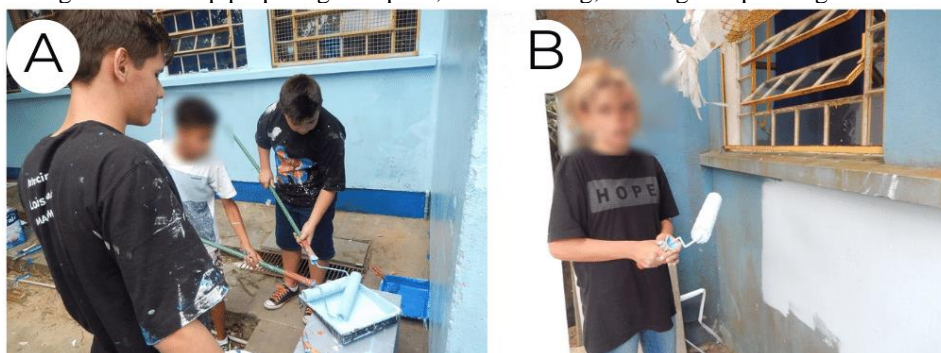
(A) Students preparing paint (B) Student painting the walls
