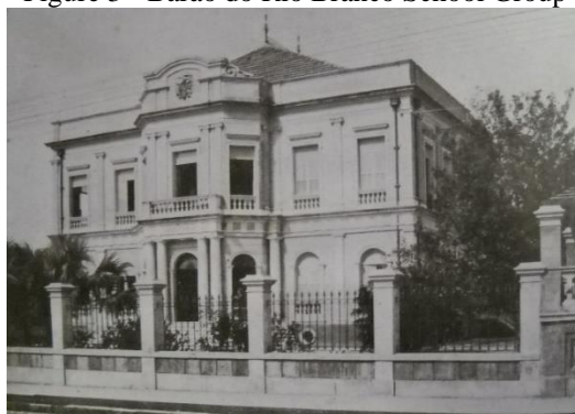
Figure 3 - Barão do Rio Branco School Group
