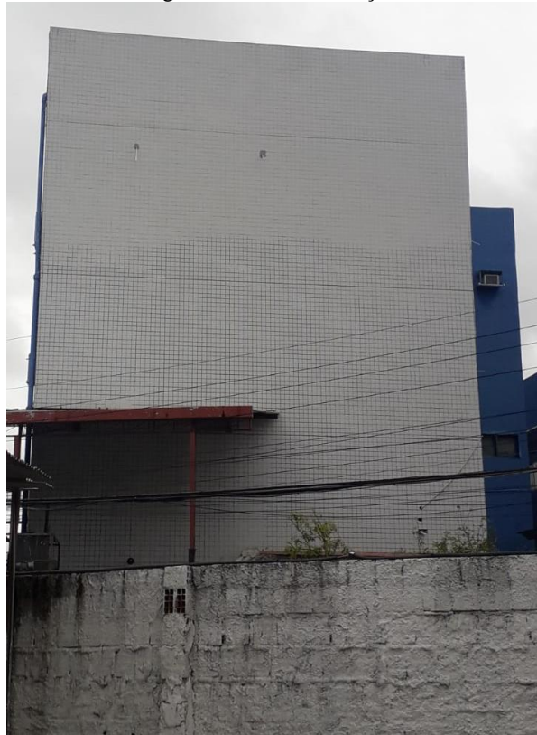
Figure 11 - Left side façade
