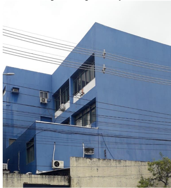
Figure 9 - Right side façade
