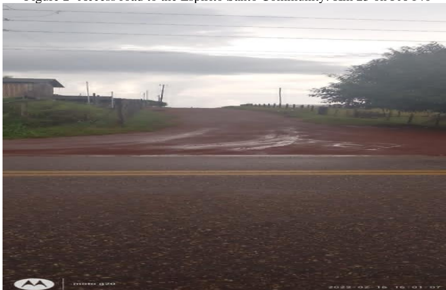
Figure 2- Access road to the Espirito Santo Community: Km 23 on PA 140
