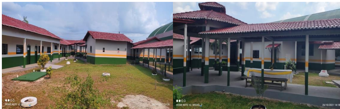
Figure 7 - a) The school has 11 classrooms and a multidisciplinary laboratory; b) Indoor covered spaces to access the classrooms.
