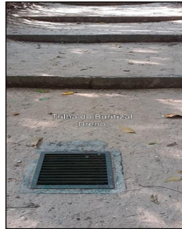
19 – Drain in the trail
