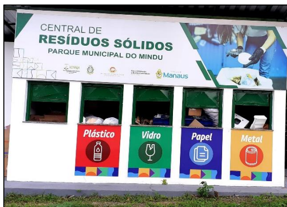
Figure 7 – Solid waste collection center
