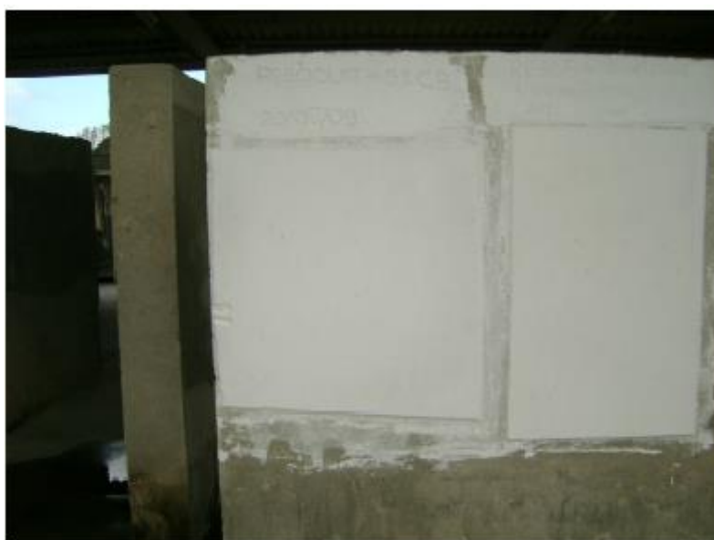
Figure 10: Coating executed with industrialized mortar with addition of CPB-40
