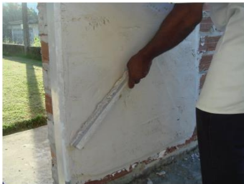
Figure 08: Mortar mortar applied directly on the masonry
