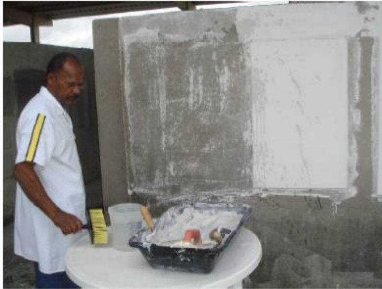
Figure 02: Base preparation for plaster application Source: ALVES JÚNIOR, 2009.
