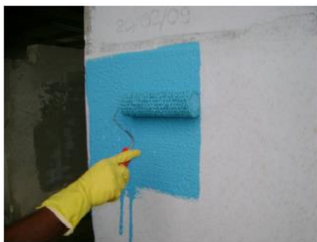
Figure 17: Execution of lime-based painting Source: ALVES JÚNIOR, 2009.
