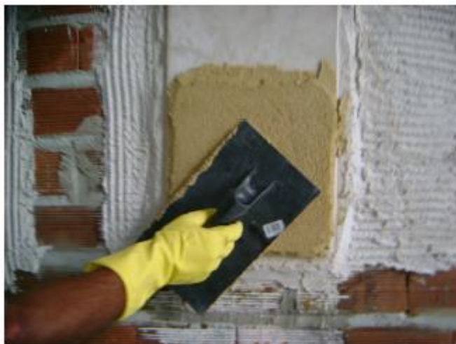
Figure 18: Finishing with a trowel Source: ALVES JÚNIOR, 2009.
