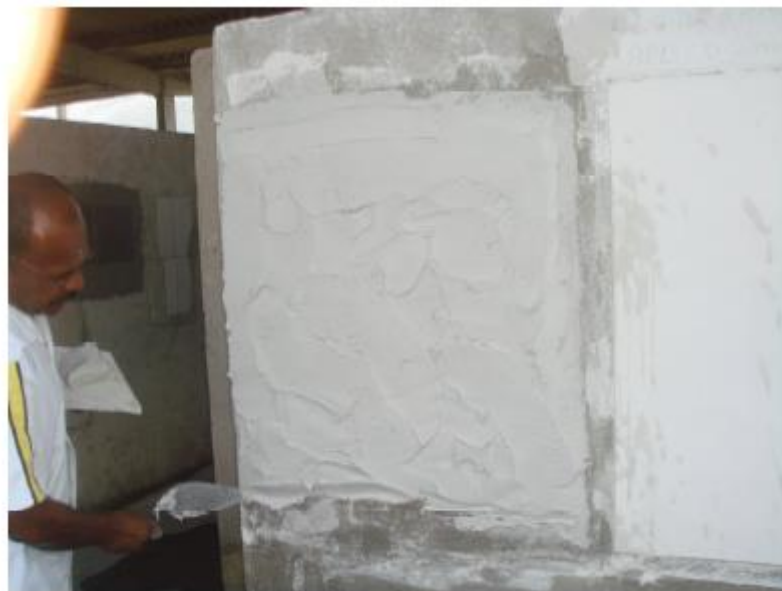
Figure 03: Application of lime mortar on cementitious substrate Source: ALVES JÚNIOR, 2009.
