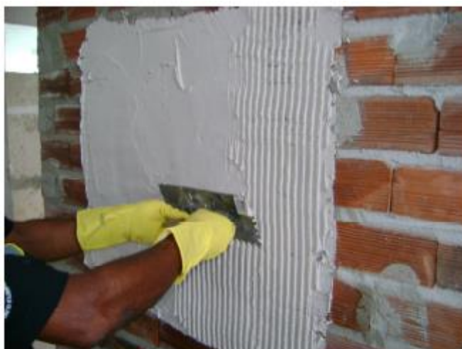
Figure 13: Execution of base preparation Source: ALVES JÚNIOR, 2009.
