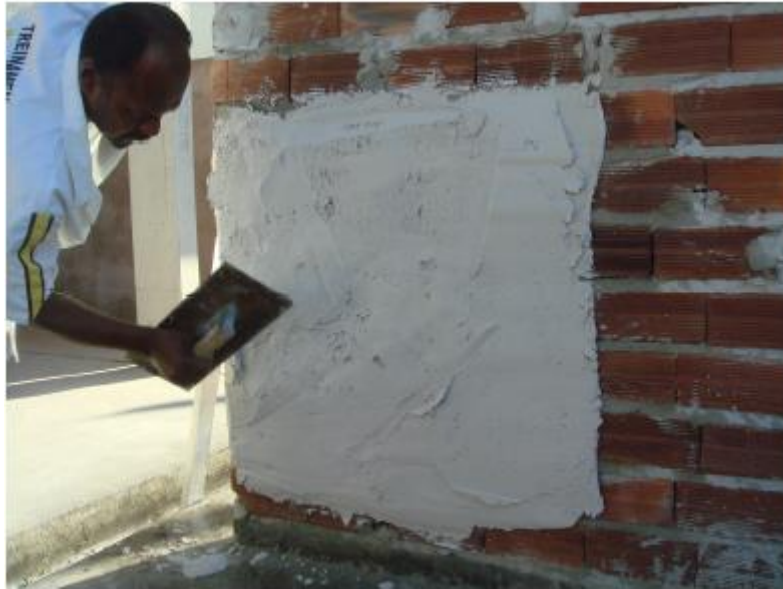
Figure 06: Direct coating application on the masonry Source: ALVES JÚNIOR, 2009.
