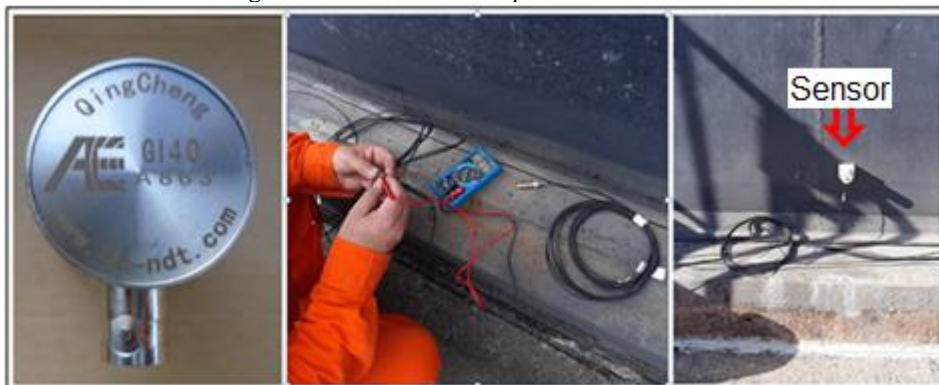
Figure 11 – Installation of piezoelectric sensors
