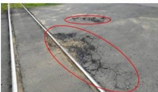
(c) Alligator leather cracks
