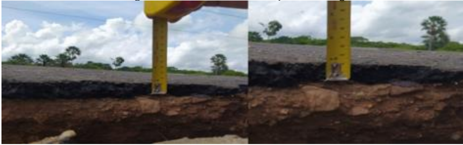
Figure 4. The thickness of asphalt coating
