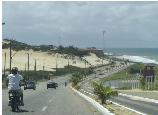
Fig. 3.4 - Coastal Way and location of the Tower considered as a reference in the measurements.
