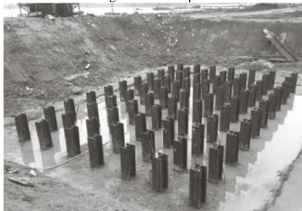
Figure 8 – Steel piles
