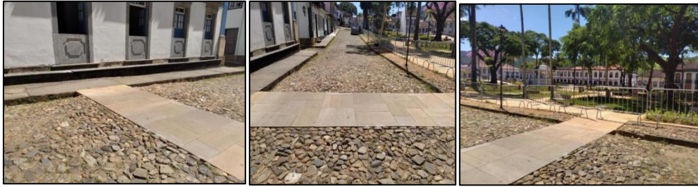
Figure 10 - Access ramp to Gomes Freire Square currently seen from three different angles
