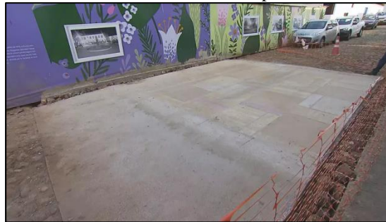
Figure 06 - First version of the access ramp to Gomes Freire Square
