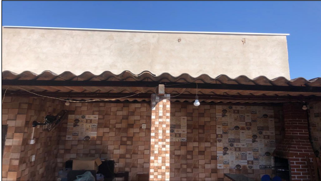
Figure 7. Roof of Implementation Analysis in Residence
