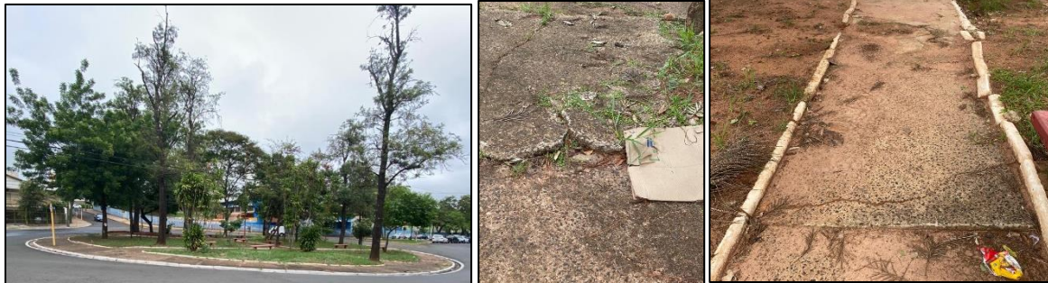
Figures 2 to 4 - Situation of the square.
