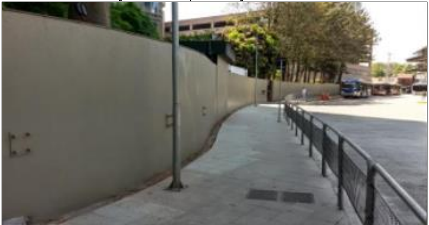
Figure 34 – Work Completed with Mega Pile Reinforcement.
