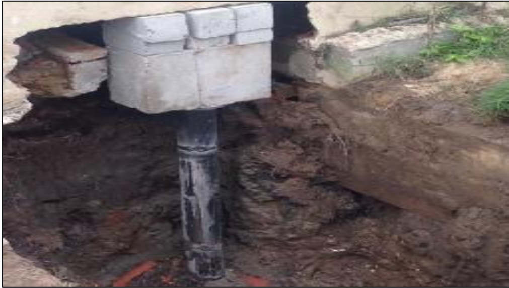
Figure 14 – Mega metal stake installed.
