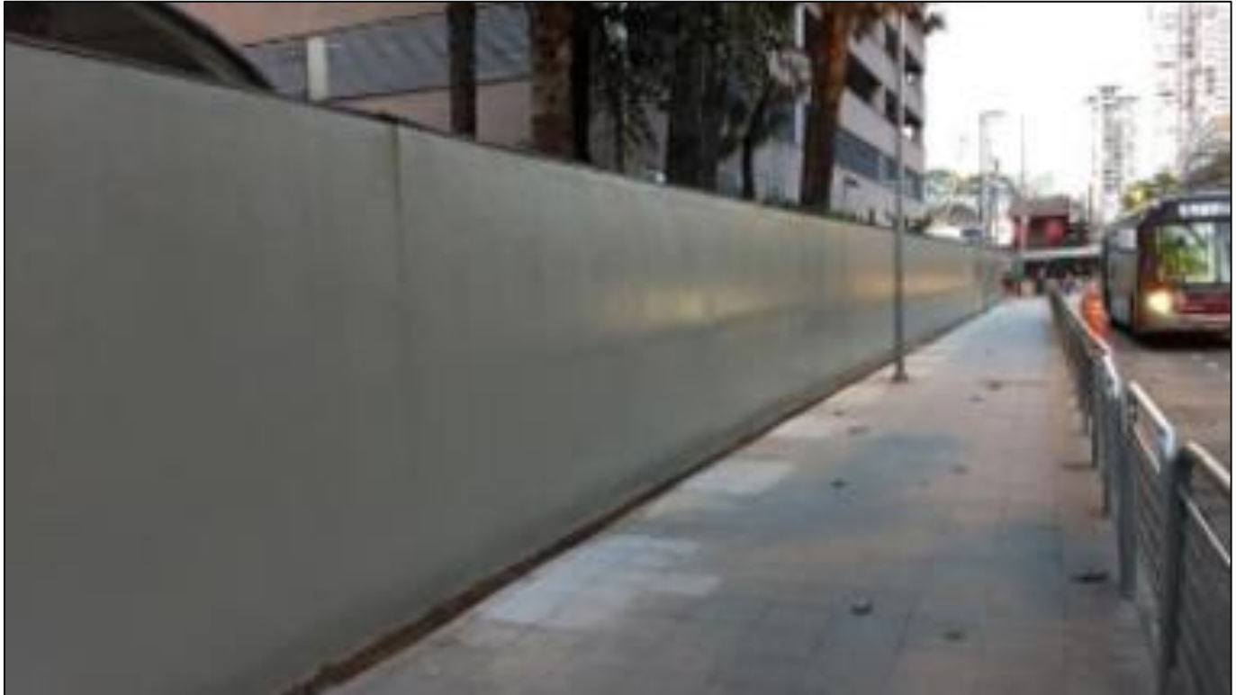
Figure 35 – Work Completed with Mega Pile Reinforcement.
