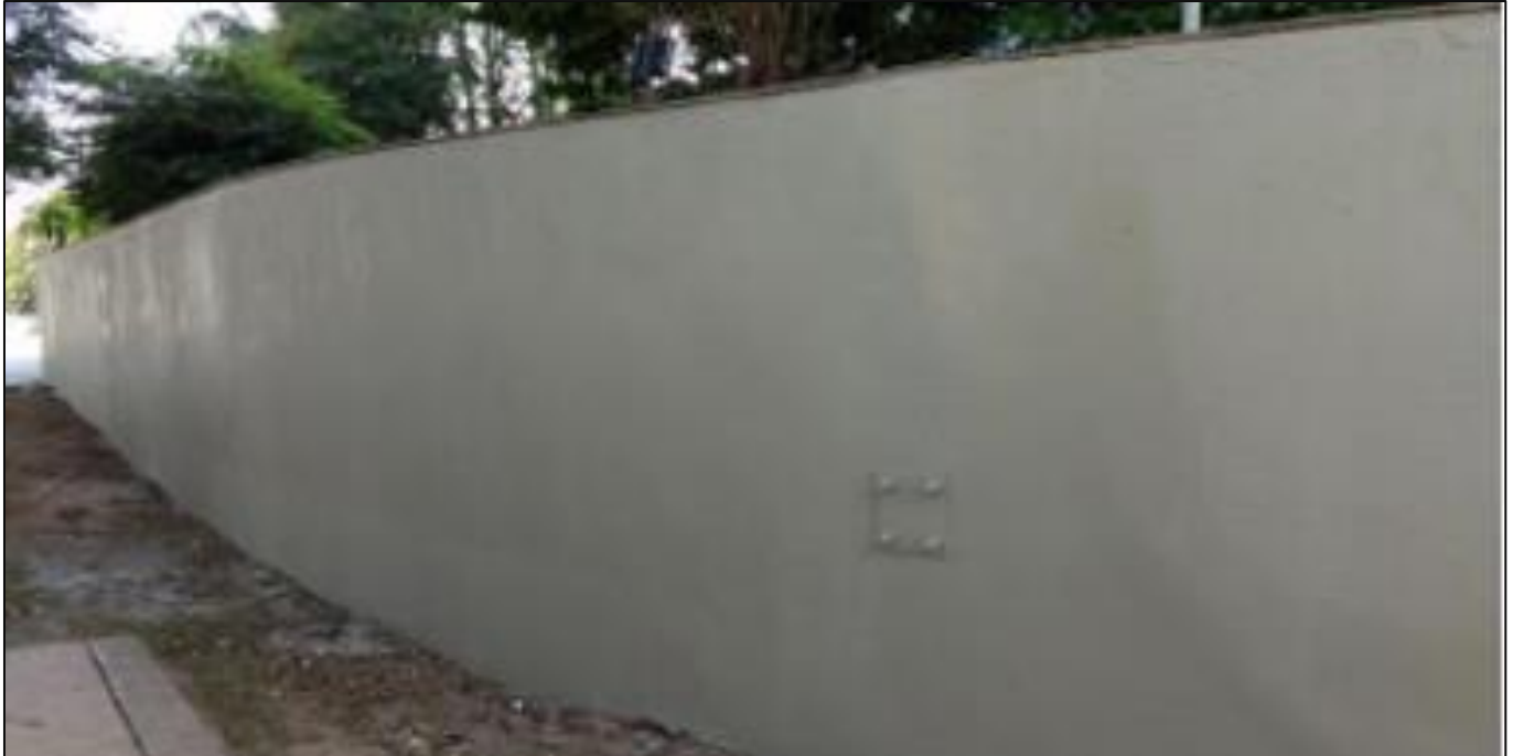
Figure 33 – Work Completed with Mega Pile Reinforcement.
