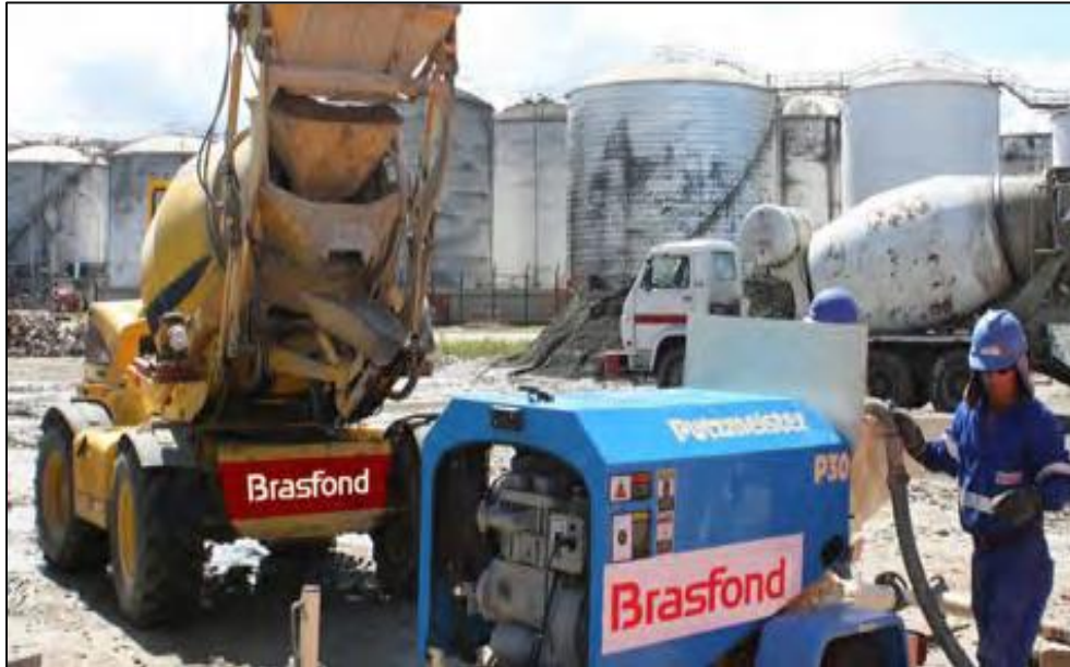
Figure 24: Concreting of the Root Pile.
