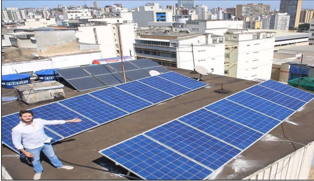
Figure 4. Installation of modules with the inclination for bifacial panels on concrete roof
