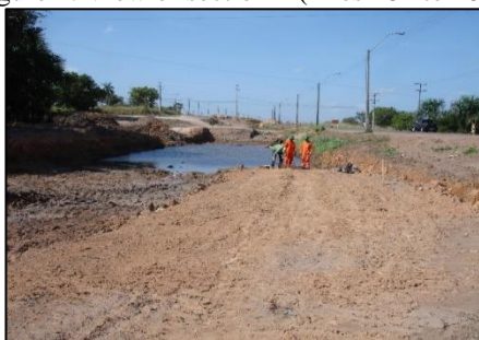
Figure 4. View of section 1 (Piles 181 to 188).
