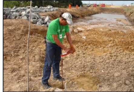
Figure 9. Preparation for carrying out the “vane-test”.
