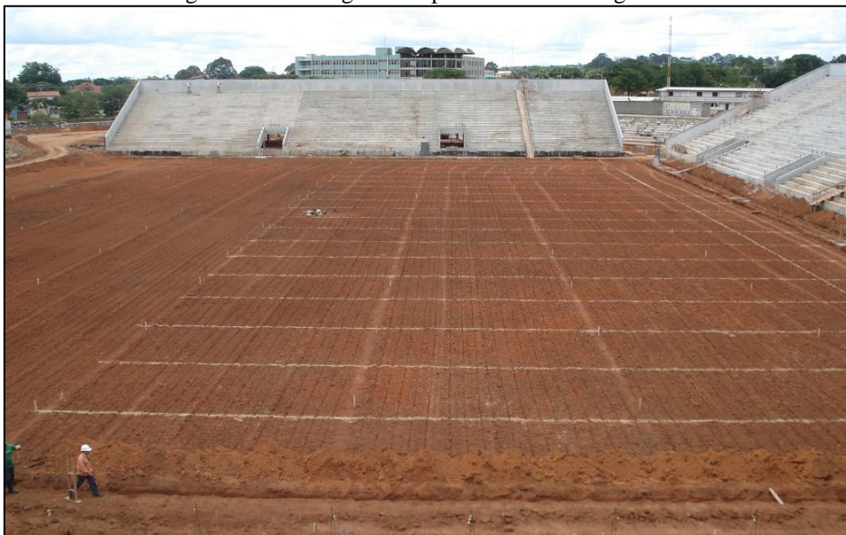
Figure 11. Marking the template for the drainage lines.
