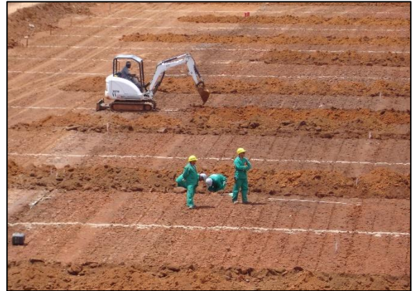
Figure 13. Opening the transverse trenches
