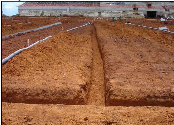
Figure 14. Trenches cleaned for installation of drainage geocomposite
