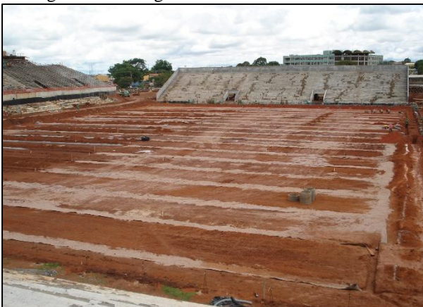
Figure 16. Filling the trenches with washed sand
