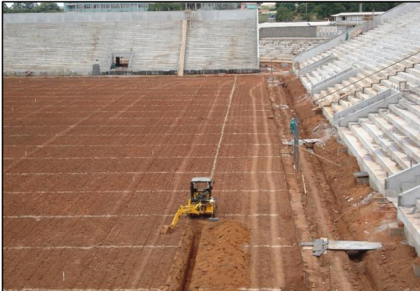
Figure 12. Opening the longitudinal trenches
