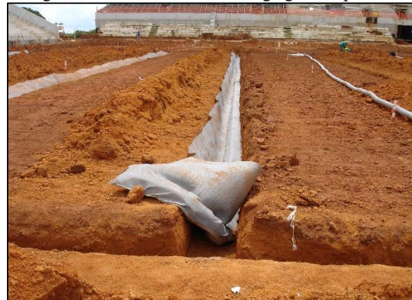
Figure 15. Installation of drainage geocomposite.
