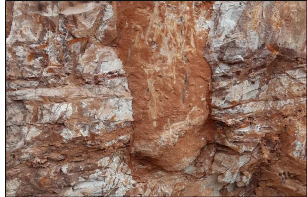
Figure 8. Continuous helix pile tip paralyzed before the expected elevation due to the strength of the material.
