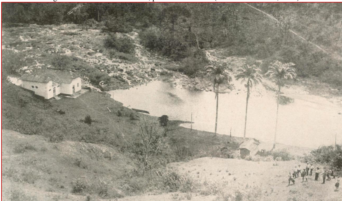
Figure 2 – Photo: Almada Plant, published in 1938. (Source: BONDAR, 1938)
