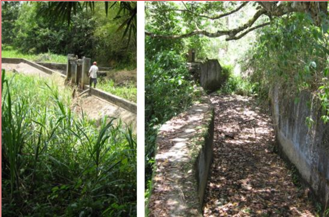
Figure 4: On the left view of the Almada Plant dam on the Bonfim Farm and on the right photo of the stone channel on the same farm. The plant's water flow was manually controlled by gear-operated gates.
