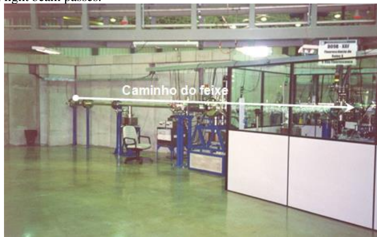
Figure 4 - Photo of the ring pipe for the DO9B – XRF line of the Brazilian Synchrotron Light Laboratory, through which the synchrotron light beam passes.
